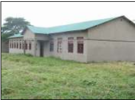
One of the four, 28 bed wards at Liwolo Hospital, Southern Sudan.
