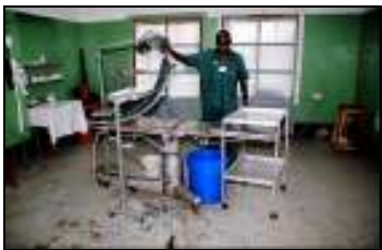
Only Operating Room in Yei
